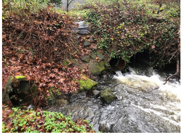
Figure 2-4: Culvert downstream of the I-405 crossing
