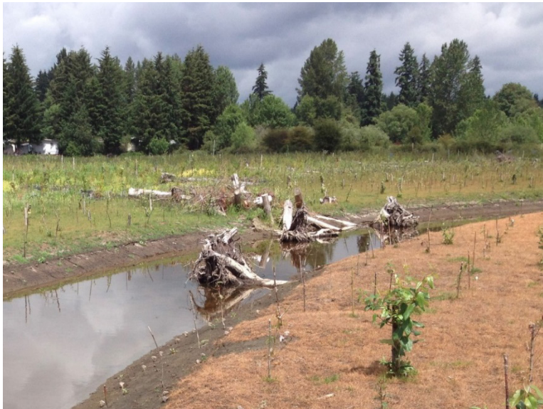
Figure 10A-2 Rootwad Habitat Structures, Evans Creek, King County
