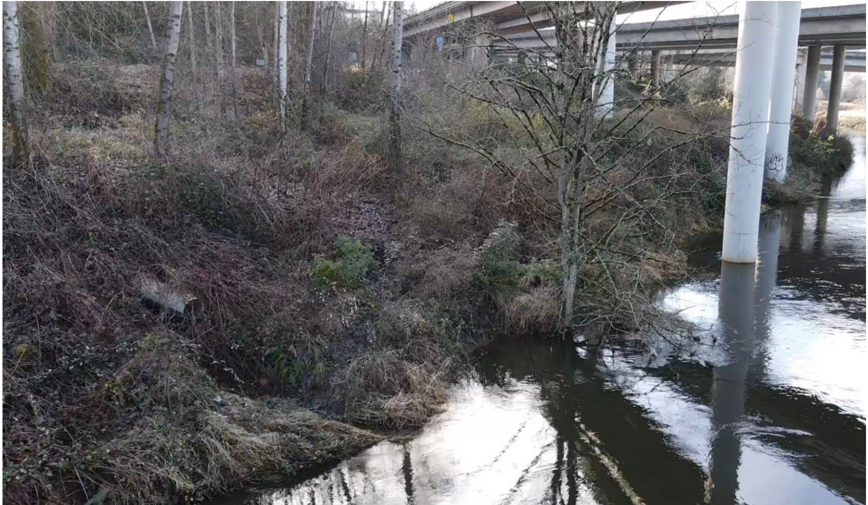
Figure 6. Photo of the Sammamish River looking west through along the south bank. Note the projecting pipe and bank scour around the existing NB I-405 ramp column (January 1, 2023 site visit).
