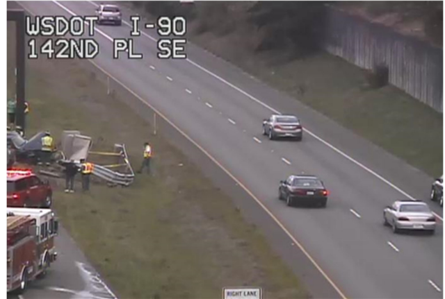
Figure 1-6: Cabinet damage due to guardrail deflection
